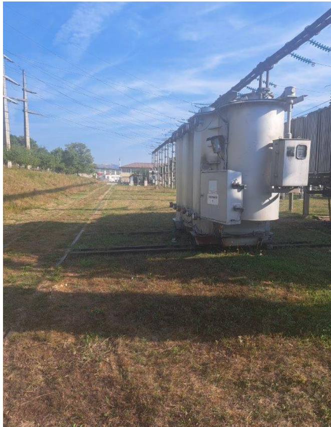
ET 110/10/35 kV nakon transporta u TS Sarajevo 1
